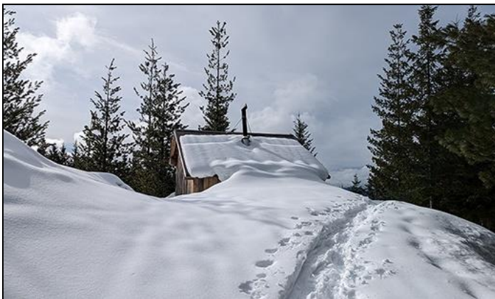
Coming up on the back side of the Maxwell South Shelter.
