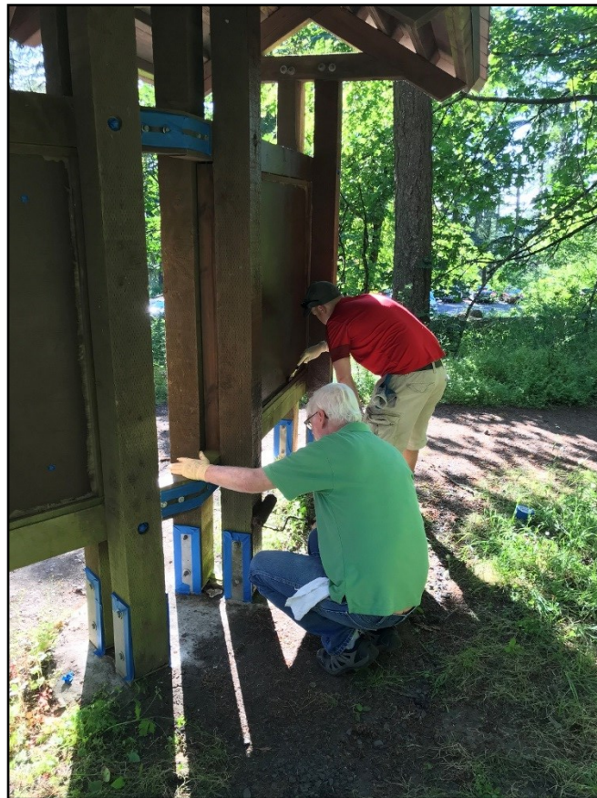
Dan and Todd put the finishing touches on the kiosk.
