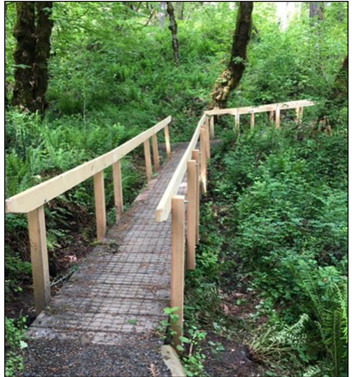
Bridge repair is complete! Photo by Janet Jacobsen.
