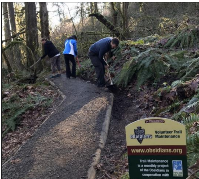
Matt, Lisa, and Jennifer work on the lower ditch.
