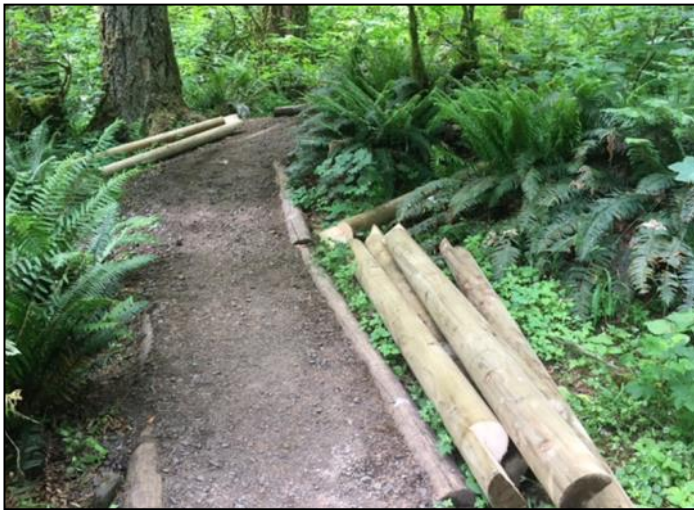
Motorized wheelbarrows were used to haul 40 plus peeler logs to replace the old ones. Photo by Janet Jacobsen.
