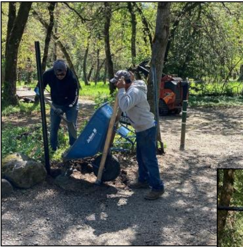
First post going in. Photo by John Jacobsen.
