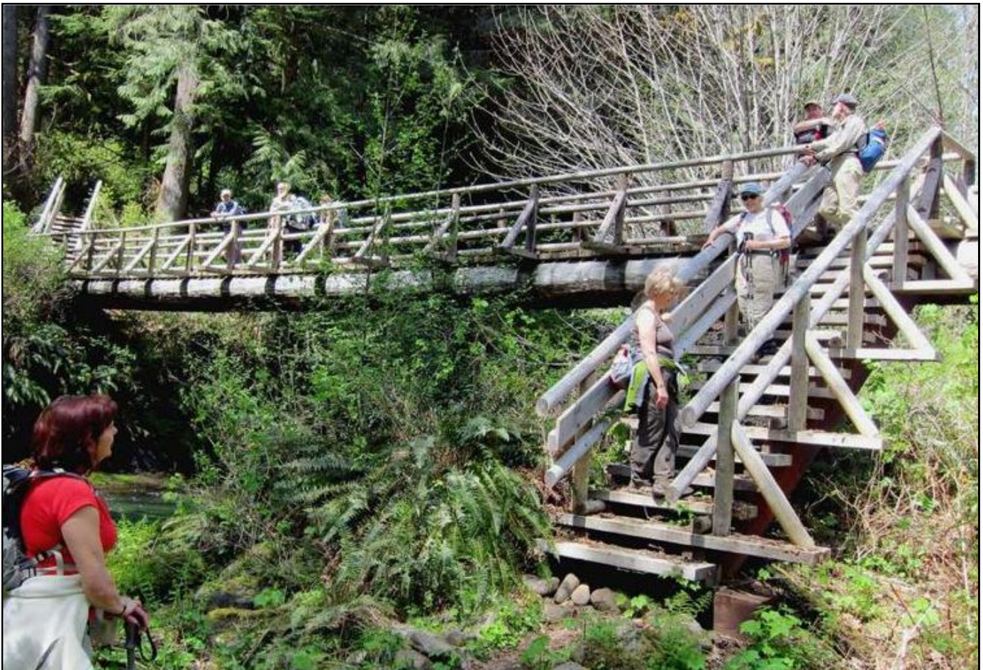
Hiking across the new bridge over the N. Fork Smith River, a big improvement over the bare logs that were there.
