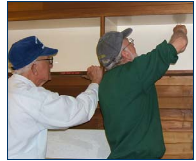
Bill and Jim removing kitchen cabinet.
